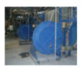
**DSC Series** The pump with the reinforced hose for high pressures. Flow-rate: up to 65 m<sup>3</sup>/h Pressure: up to 15 bar.
