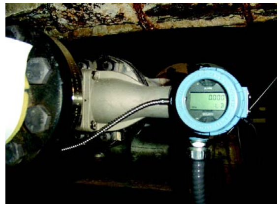
We Energies' Rosemount 8800D MultiVariable steam installation.
