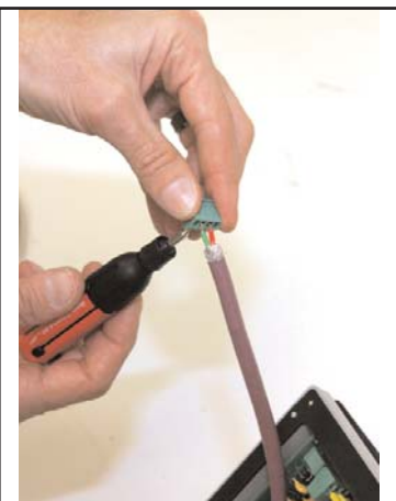
Wiring Profibus cable to 4-lead terminal block
