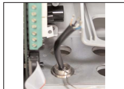
M12 adaptor cable assembly secured to grounding plate.
